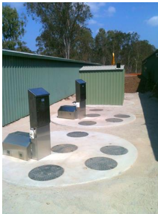
Figure 4 Example of an installed 10kL/day STP (Courtesy of Taylex)
